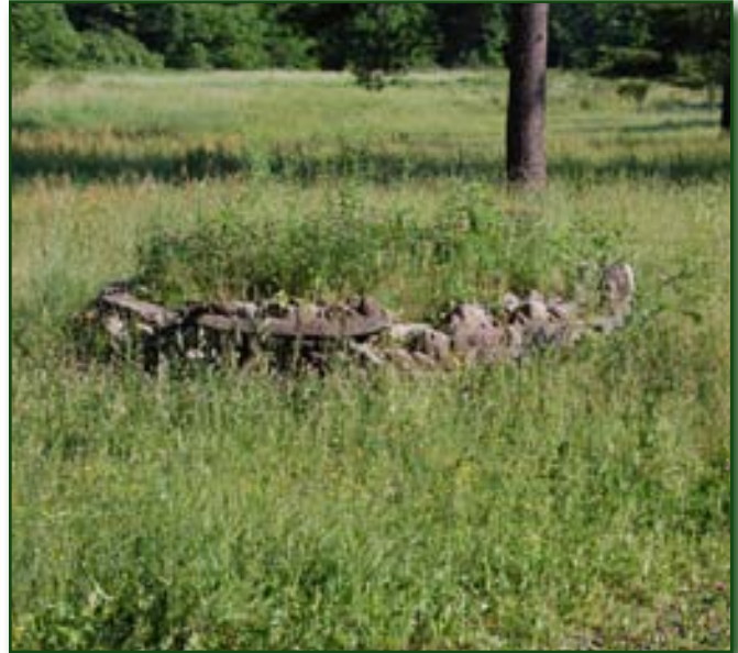
Before: Tall grass and overgrown weeds obscure the beauty of the stone work of what will soon be transformed...
